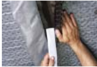
Integrated self-adhesive tape for laying precision.
