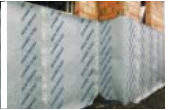
Permanent filtration and drainage.
