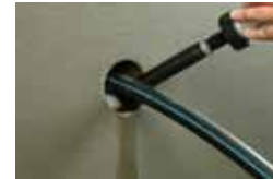
2. ... pipe is sealed...
