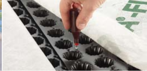
Joining sheets with DELTA®-FLORAXX connecting elements.
