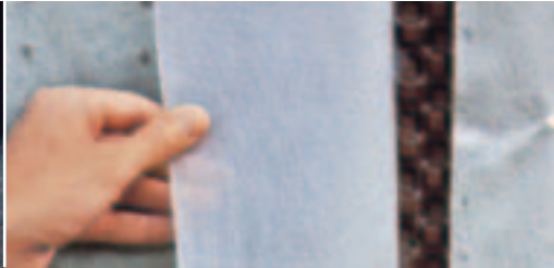
Edge overlap of dimpled sheet and geotextile.
